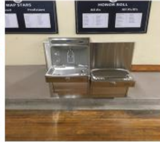
3. Newly Installed Fountain at Fanning Middle
