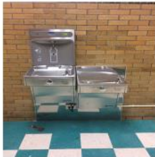
1. Newly Installed Fountain at Gallaudet
