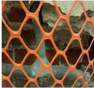
1. Lead Crossover Pipe
