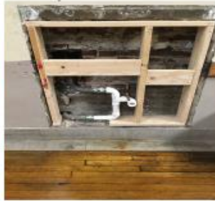
2. Framing for Replacement
