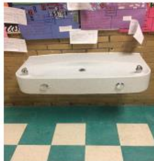
2. Newly Installed Fountain at Gallaudet
